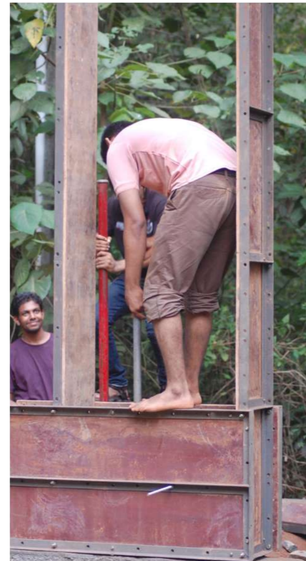
RAMMED EARTH CONSTRUCTION
