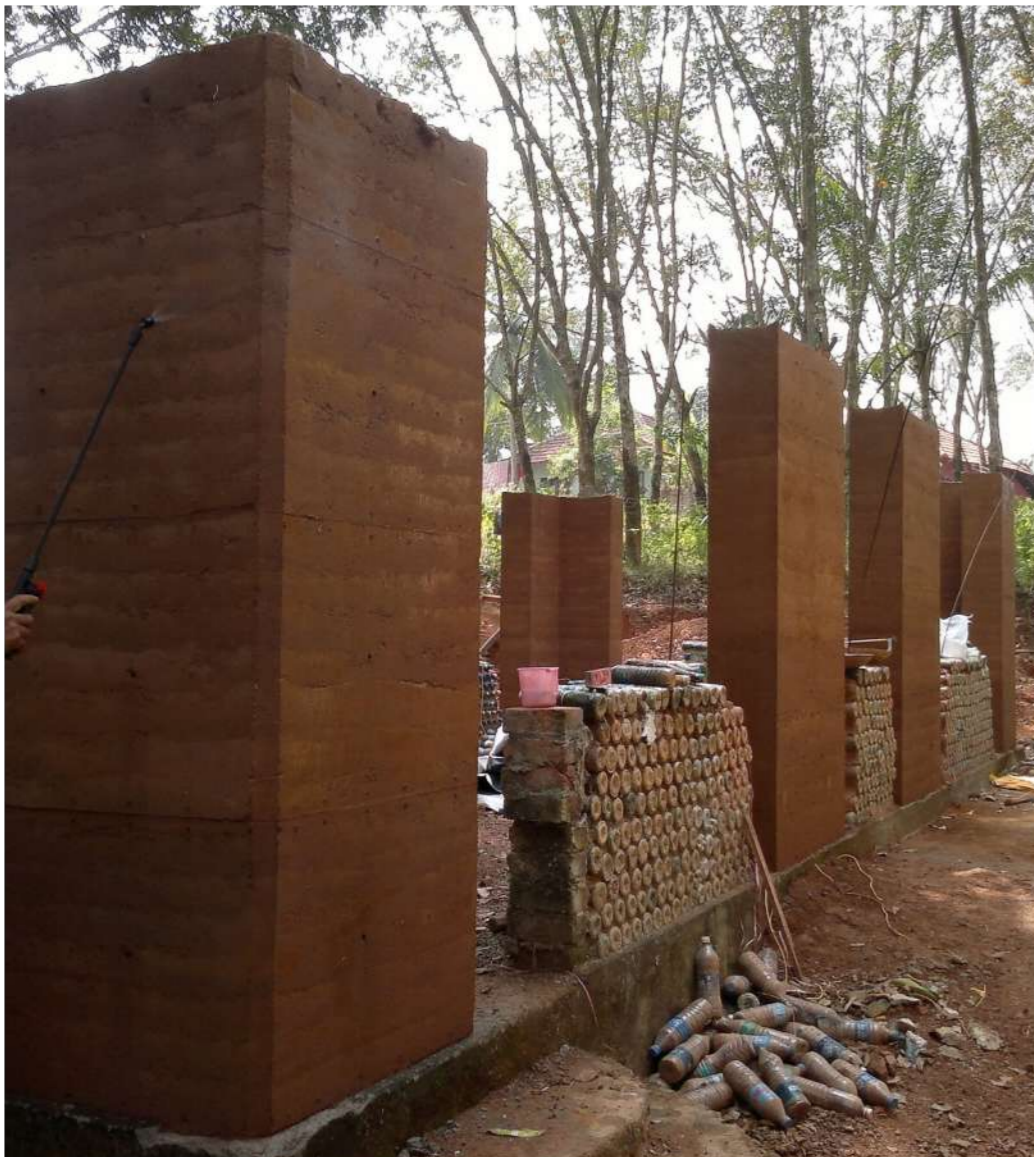
RAMMED EARTH WALLS & BOTTLE WALL WITH USED PLASTIC BOTTLES
