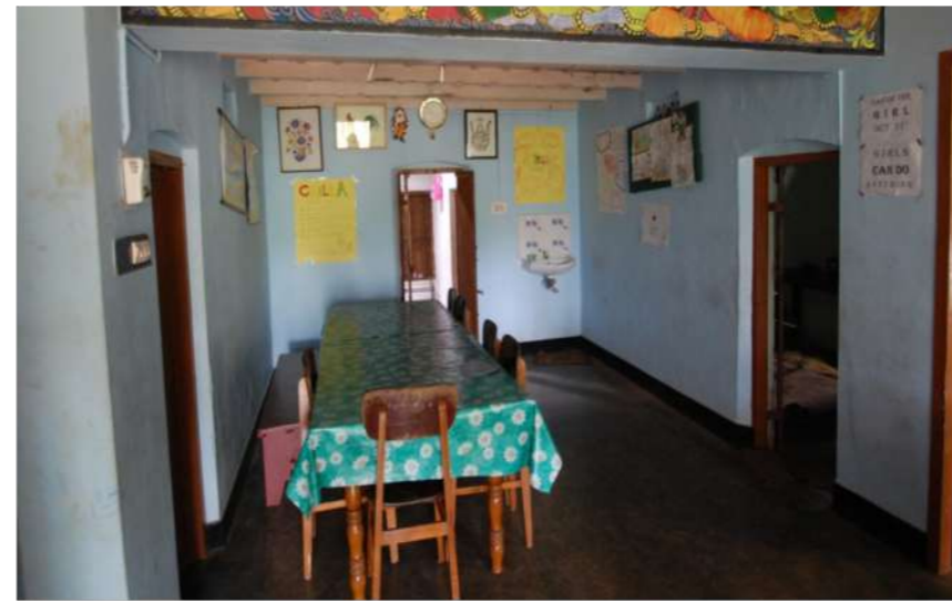
EXISTING DINING ROOM
